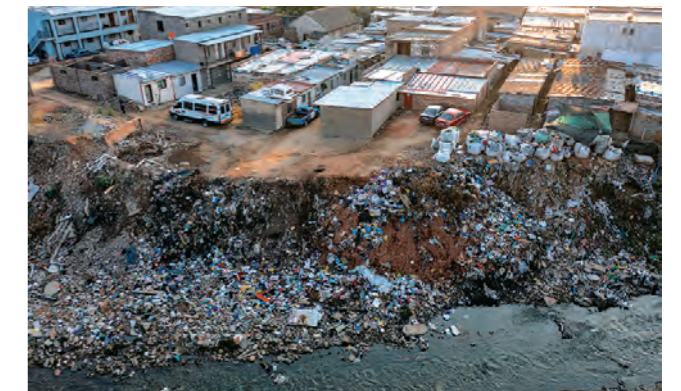
Waste problems in South Africa. Garbage that exceeds disposal capacities is dumped on the outskirts of some cities, polluting soil and water.
