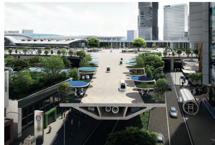
Illustration of the sky deck that connects the various zones. A pedestrian sky deck will be installed above the roads where private cars and traditional public transport operate. Short-distance travel will be supported by small, self-driving electric vehicles.
