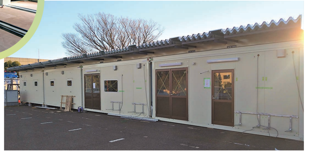
In hospitals lacking ICUs, medical containers are set up on the premises and used as hospital wards. The photos show a prefabricated ICU ward and its interior, which were preliminarily assembled in Japan. After this, it will be installed in a hospital in Kenya.
